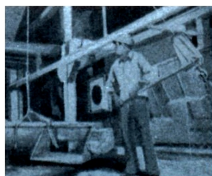
Conveyor being lifted into position with ABLE WRP.
