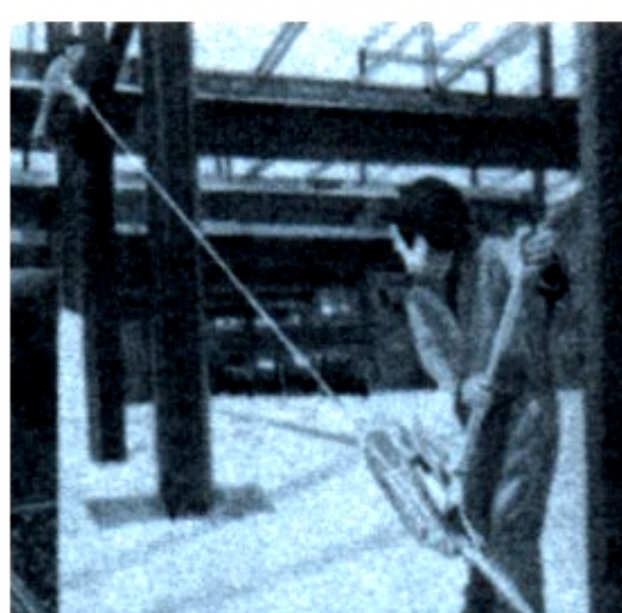
ABLE WRP used for steel alignment during erection.
