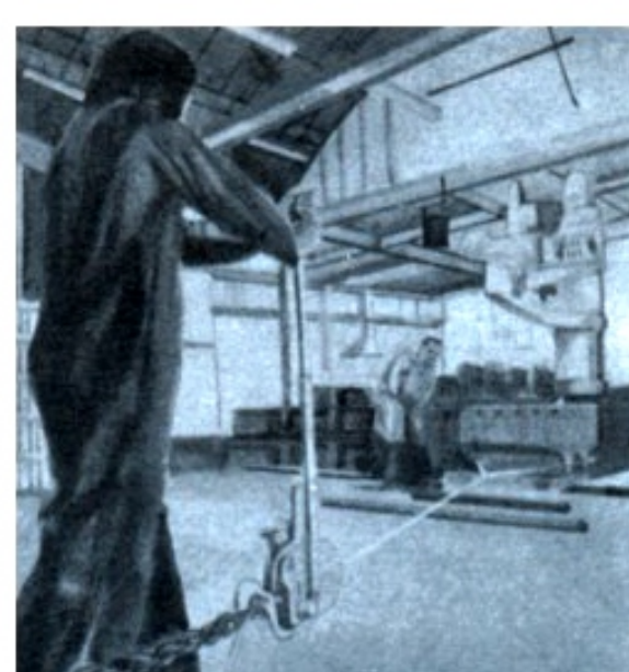
ABLE WRP in operation for the positioning of heavy machinery.
